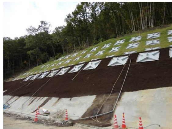
Fig. 9 Anchor & biotechnical slope protection
