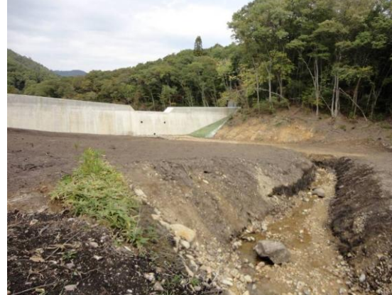
Fig. 7 Upstream view of a concrete check dam
