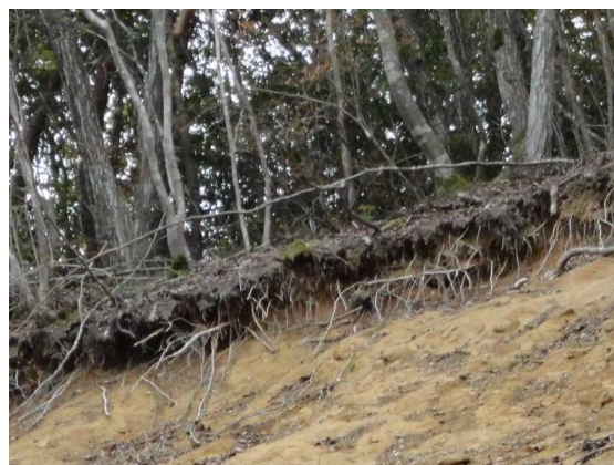
Fig. 3 Topsoil layer located on the upper part of slope
