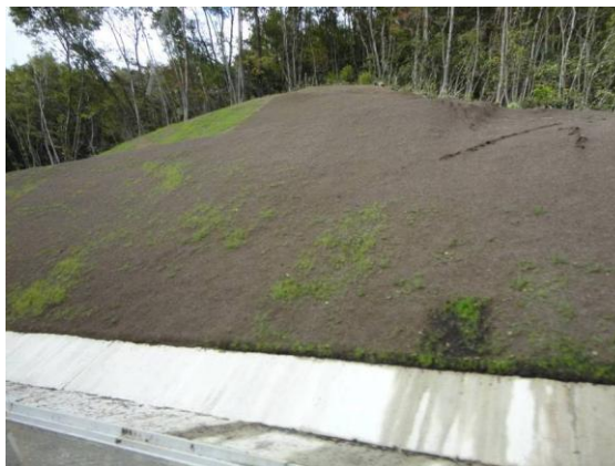
Fig. 8 Biotechnical slope protection
