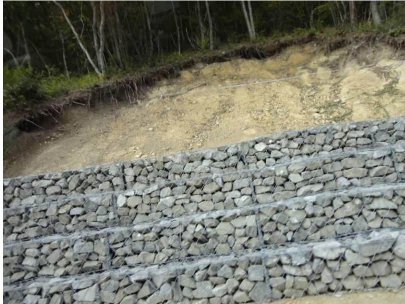
Fig. 10 Gabion wall along the road
