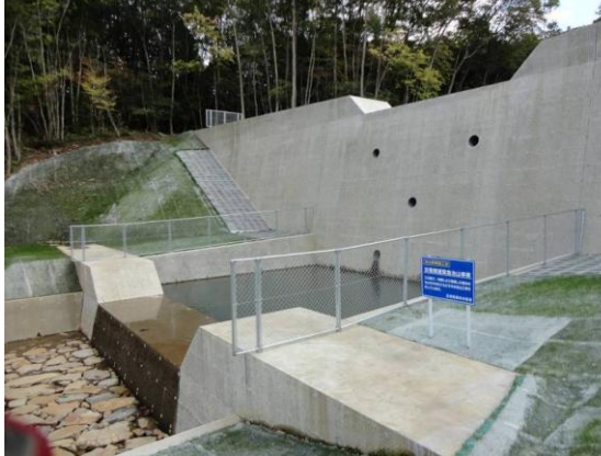
Fig. 6 Concrete Check dam with low-flow center section
