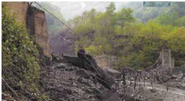
Fig. 6 The suspension bridge that was completely destroyed by the May 2004 debris flow in the Bettou-dani (Photo courtesy of the Kanazawa Office of Rivers and National Highways, MLIT)
