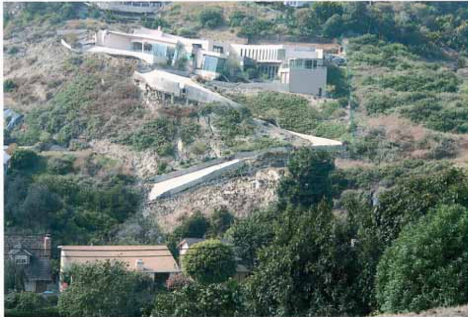
06-02-05 Bluebird Landslide of 06-01-05 GEOFIRM
