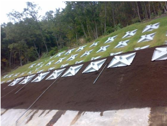
Figure 6 Bolted Anchor structure
