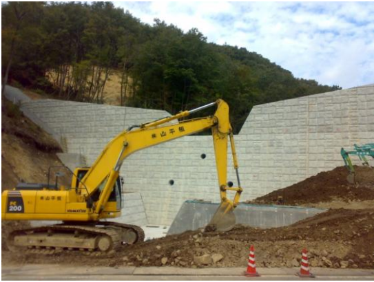
Figure 5 Sabo dam structure
