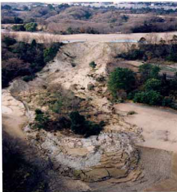
Fig. 3 Picture of the Takarazuka landslide that followed the Great Hanshin earthquake of 1995.
