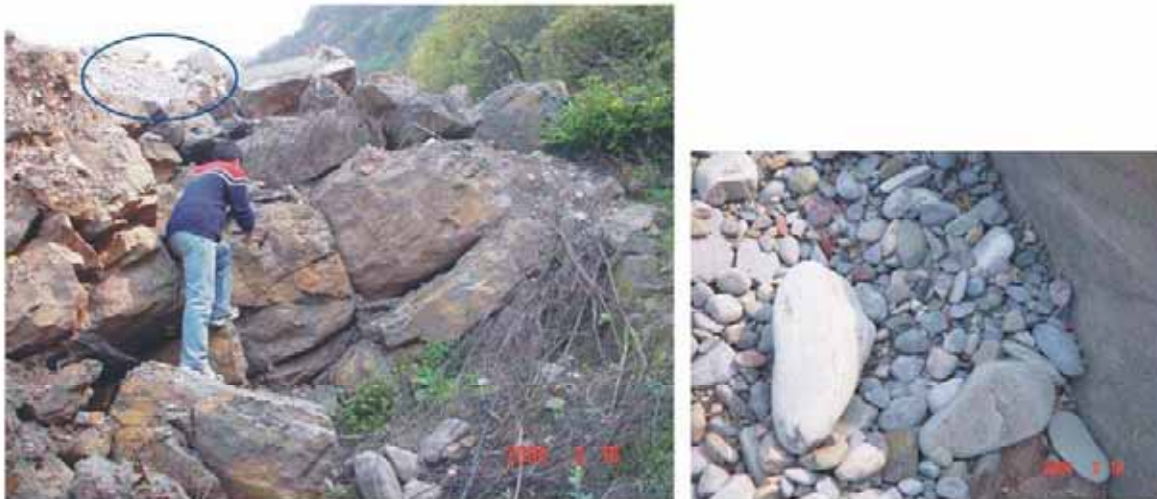
Fig. 7 Gravels displaced from the bed of Qinggan-he River and deposited in the toe of the landslide deposit (circled in photograph). Note that the sandstone dip direction is reversed and the dip angle has become steeper compared with Figs. 4 and 5)
