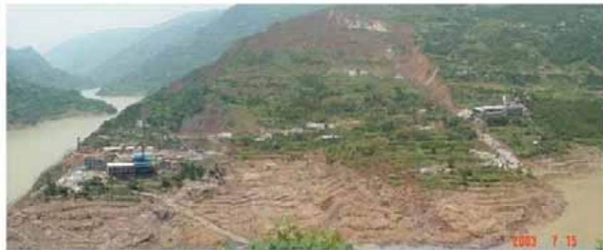
Fig. 3 Front-on view of the Qianjiangping landslide (taken by YM Zhang, July 15, 2003)
